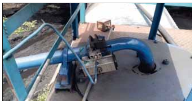
Fig. 4.1.2 : Level transmitter and control valve for the water storage tanks
