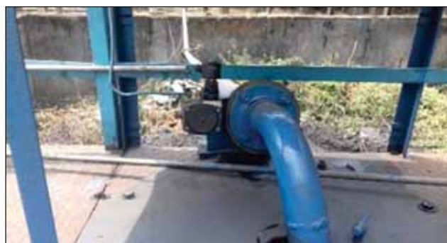
Fig. 4.1.2 : Level transmitter and control valve for the water storage tanks
